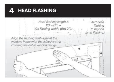
Wipe the head flange, jamb flashing and sheating with a clean rag. Cut the head flashing to twice the width of the rough opening + 2x the width of the flashing plus 2". Install the head flashing by pressing firmly in place in one direction to prevent voids.
